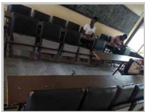
Room 37 before Renovation
