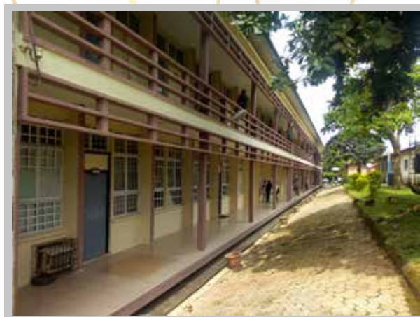
Faculty Annex Building
